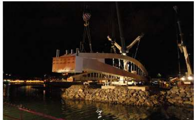
Fig. 10: Erection of the first arch
