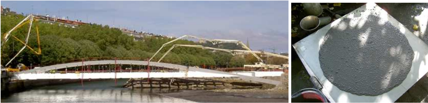
Fig. 11: Filling of the arches and test of the concrete.
