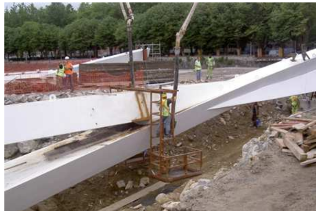
Fig. 8: Filling the arches.
