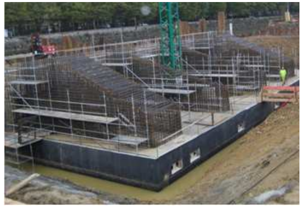
Fig. 6: Works in the abutment.
