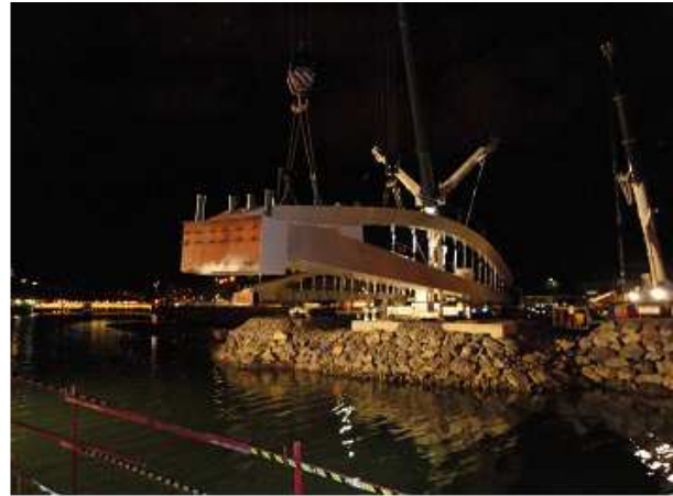
Fig. 2: Erection of the first arch.
