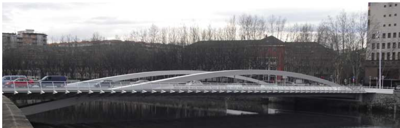
Fig. 1: Elevation from downstream.
