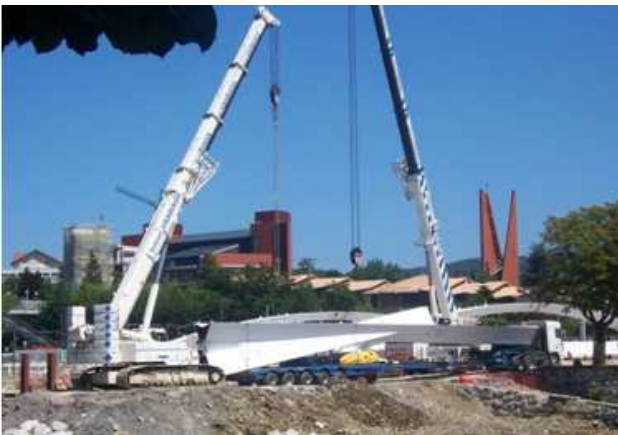
Fig. 7: Lift of the first segment.
