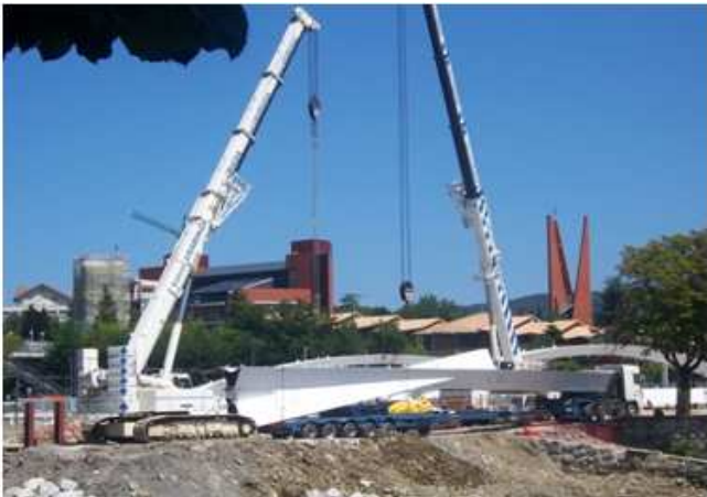
Fig. 3: Lift of the first segment
