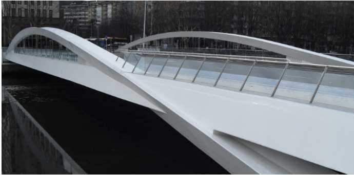
Fig. 3: Arches and the central joint.
