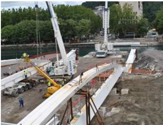
Fig. 9: Assembling of the arches.
